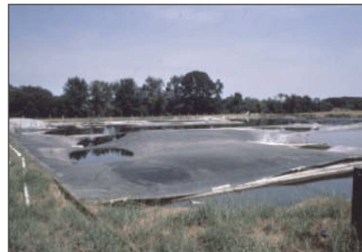
Plug Flow and Covered Lagoon Digesters
