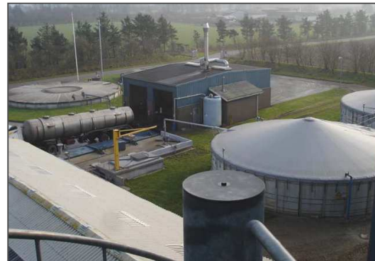
Complete Mix Digesters
